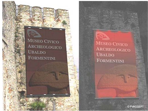
Picture 4: Solar information board in La Spezia / Italy; listed monument; realized PV demonstration project
