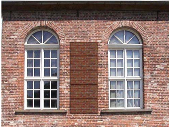
Picture 3: PV facade installation in Putbus / Germany; building under monument protection; not realized
